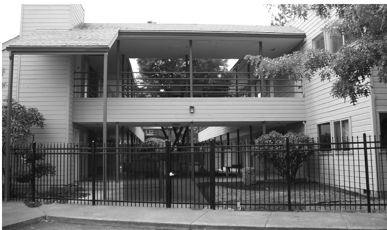
(Left) Front Gate and Courtyard
